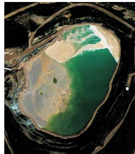
Old Rabbit Lake Open Pit Mine with tailings from the mill
